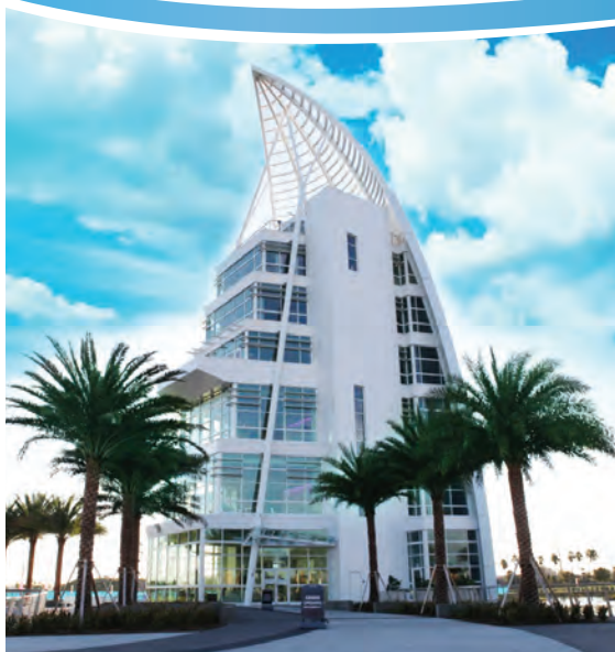
Exploration Tower at Port Canaveral
