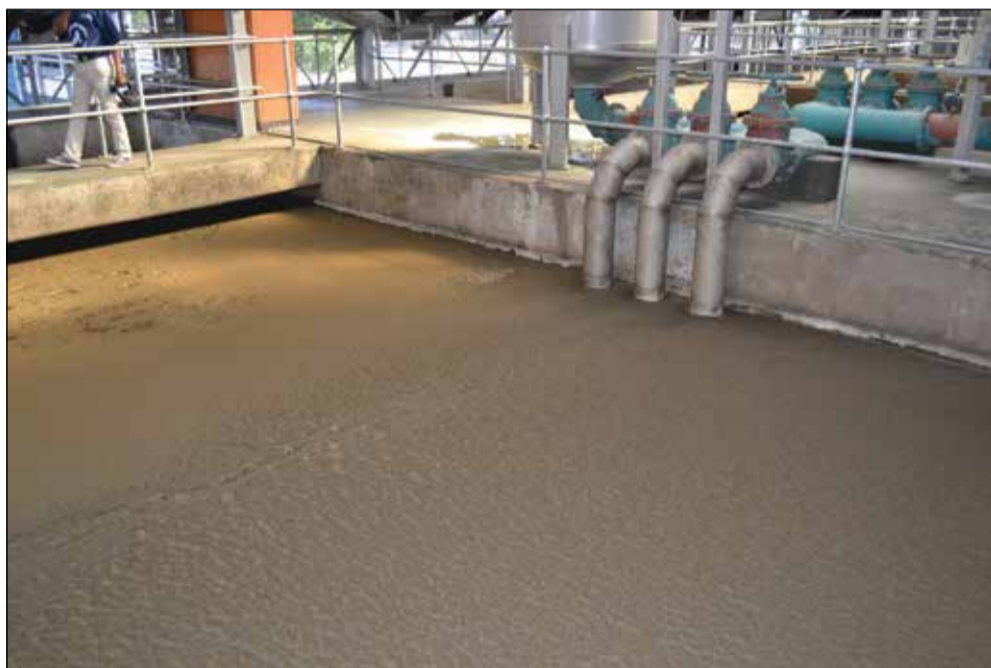
The solids removed from the water at the Brits water treatment plant.
