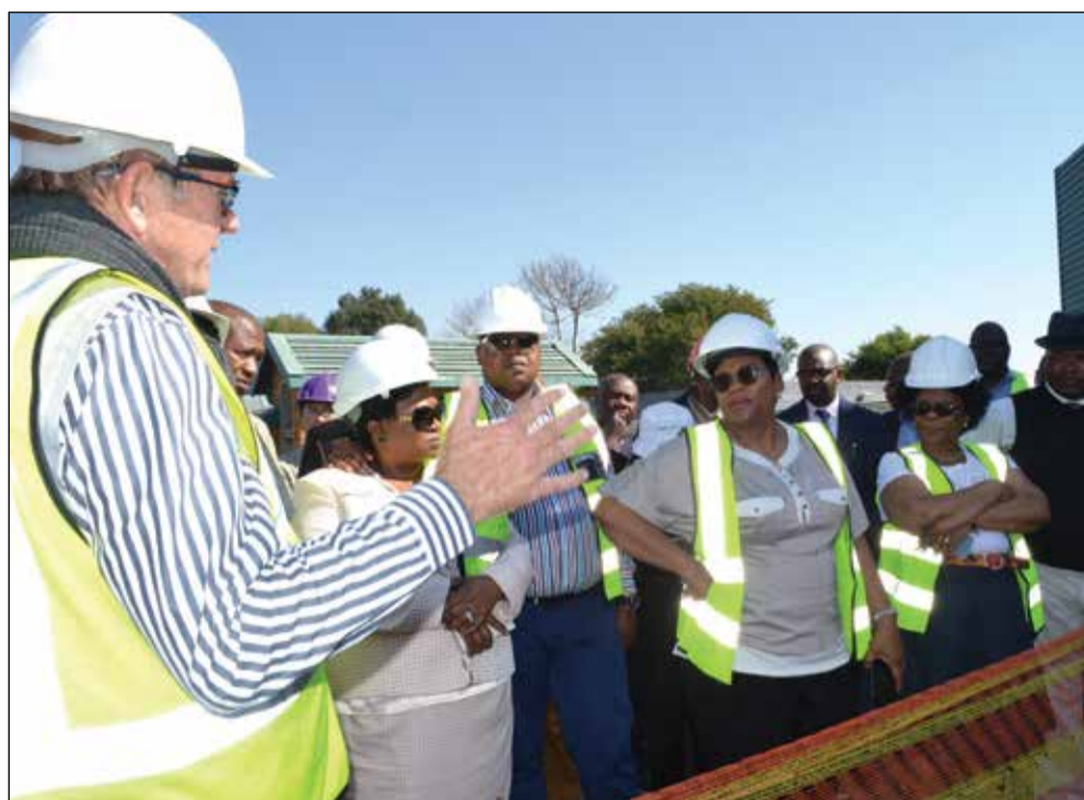
Trevor Balzer from the department of water and sanitation explains the upgrading of the Brits water treatment plant to minister Nomvula Mokonyane.
