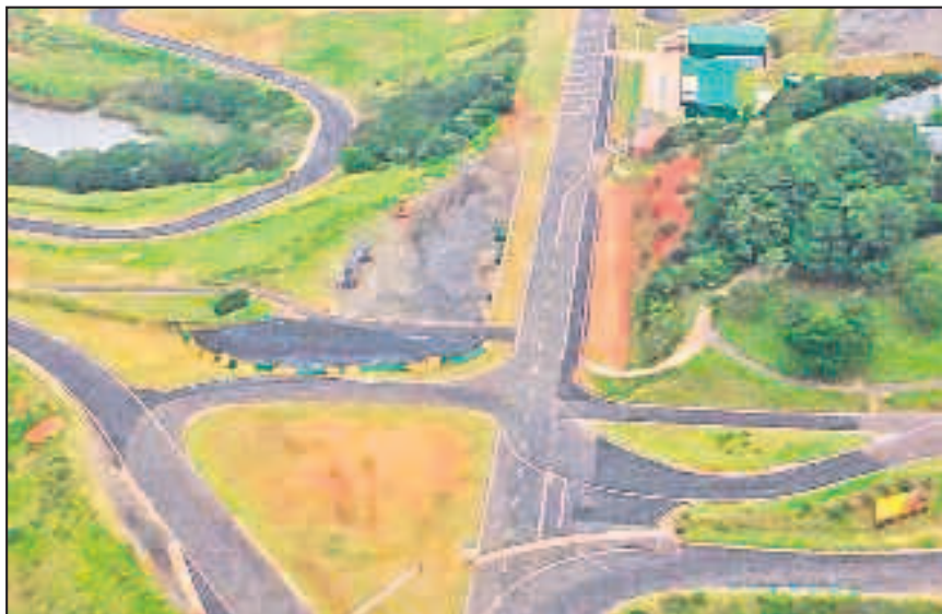
The new drag strip forms part of a larger race facility at the Dezzi Raceway in Port Shepstone.
