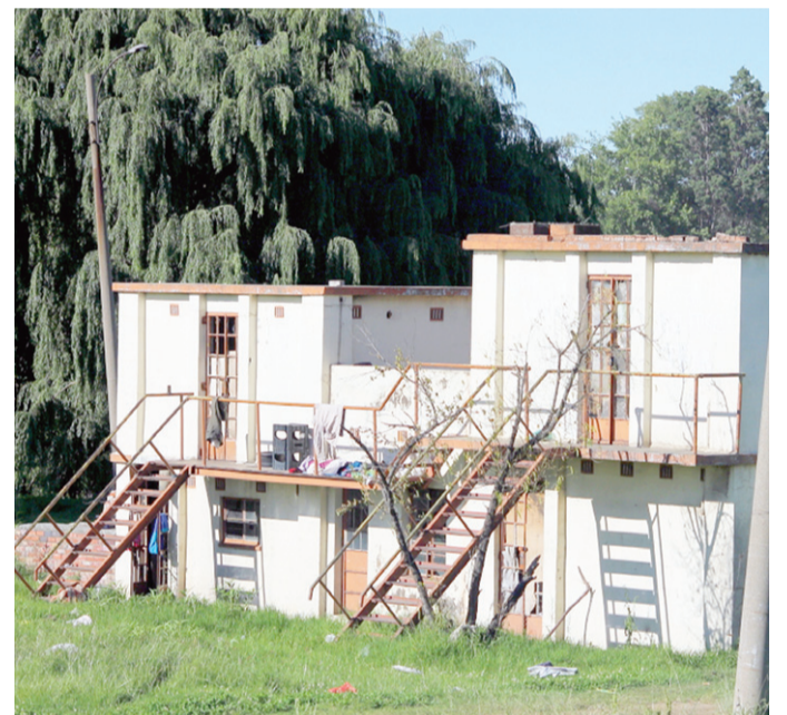
The abandoned municipal building next to the N17 highway.
