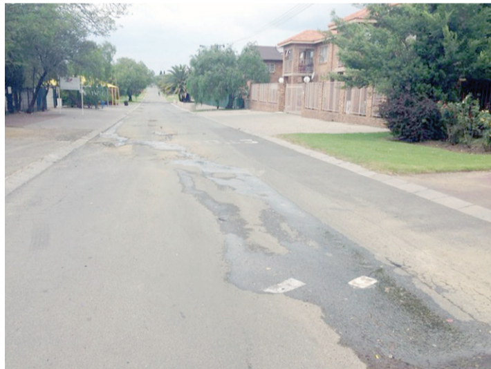
Sewage is a huge concern in Trichardt.
