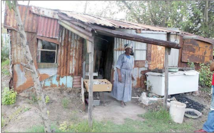
Ms Emmelina Nkosi says her home is the only one in the street that does not have water and electricity.
