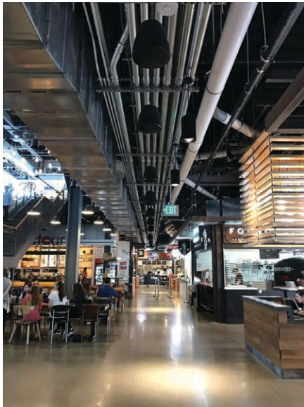
Pendant speakers on each floor deliver even levels of high-quality audio throughout the Food Hall.
