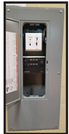
A wallplate with wall panel button control processor enclosed in an electrician-supplied protective cabinet.
