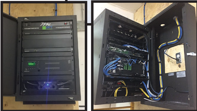
The AV rack, with cable management, mounted inside the wall at the Wiinibekuu School gym.
