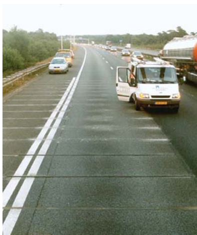
Multiple-sensor weigh-in-motion site in the Netherlands
