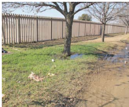
Another leaking manhole in Oliver Tambo Street in Secunda.
