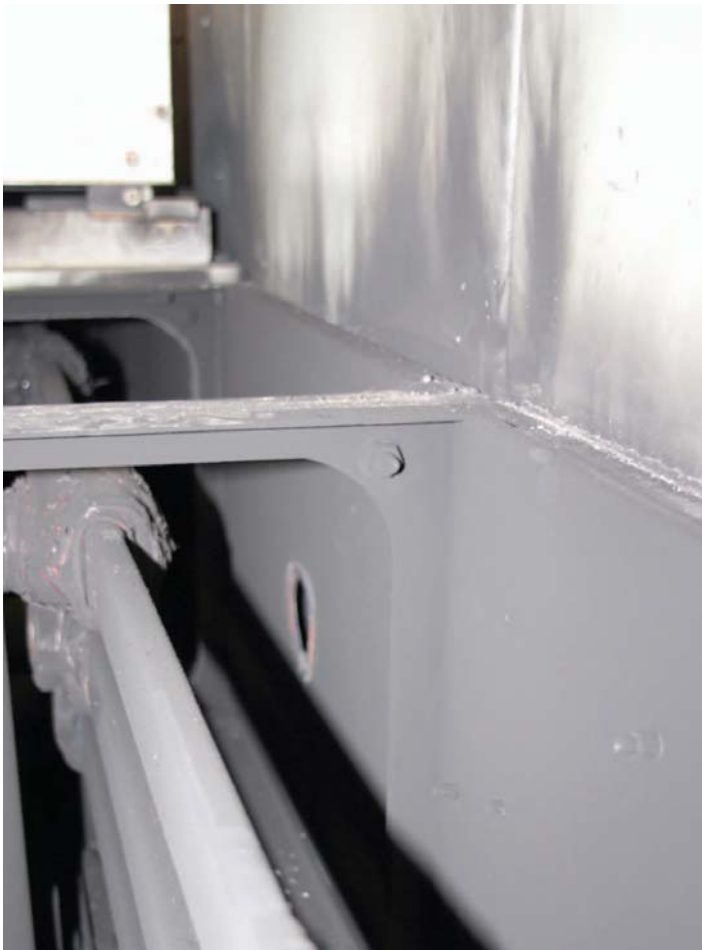
The busbar burned out. On the right side is a hole that was caused by the explosion.
